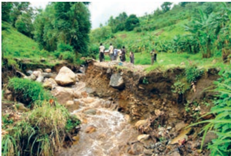
Erosion at the Mpanga River. Photo: The Niles / Henry Lutaaya
